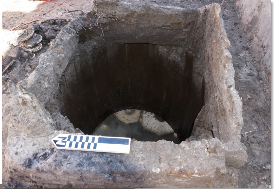
Above: Barrel well; white sand at the bottom is fanning out as fresh water flows in.
